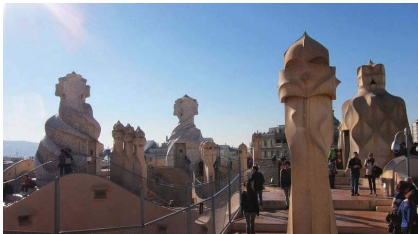
Chimneys of La Pedrera
